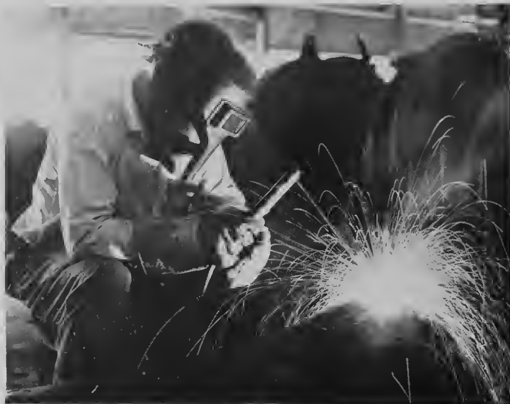
HOT SPARKS, intense glare are no friends of Lago's welders. Working safely to these employees means wearing a face shield with special glass and welder's gloves. A hard hat completes the protective gear.
